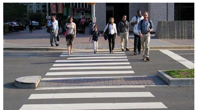
Figure 4.32 Clearly marked cross walks and pedestrian refuge islands are important for pedestrian safety and vehicular awareness of pedestrians.
