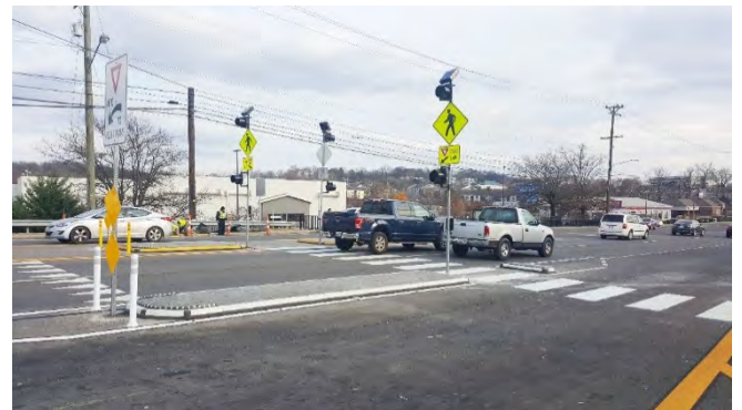
Figure 4.31 A new mid-lock crossing on 12 th Avenue South, like this one on Nolensville Pike, may be an enhancement to help pedestrians safely cross 12 th Avenue South.
